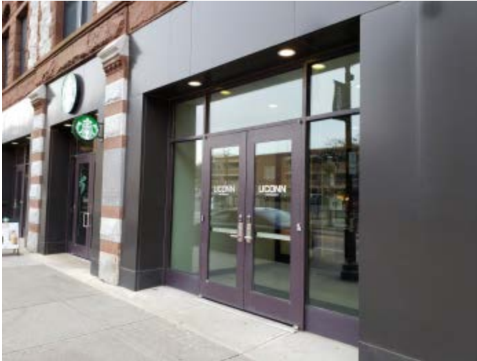
Waterbury Rectory Building Main Entrance
